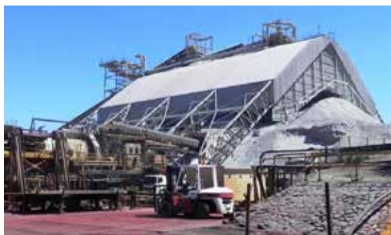
Figure 19: Fine ore stockpile
