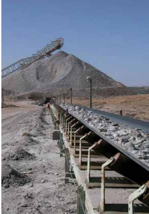
Figure 5: Coarse ore stockpile and coarse ore reclaim conveyor
